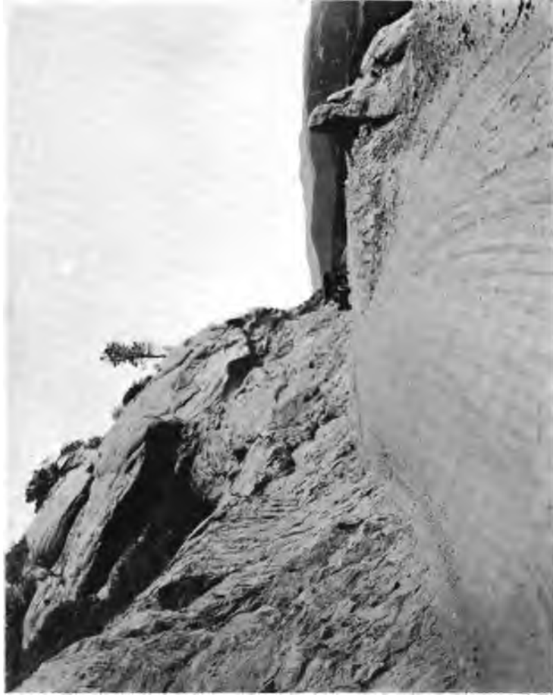
Wide roadways in the mountains form part of the "safety" plans of the California Highway Commission.
